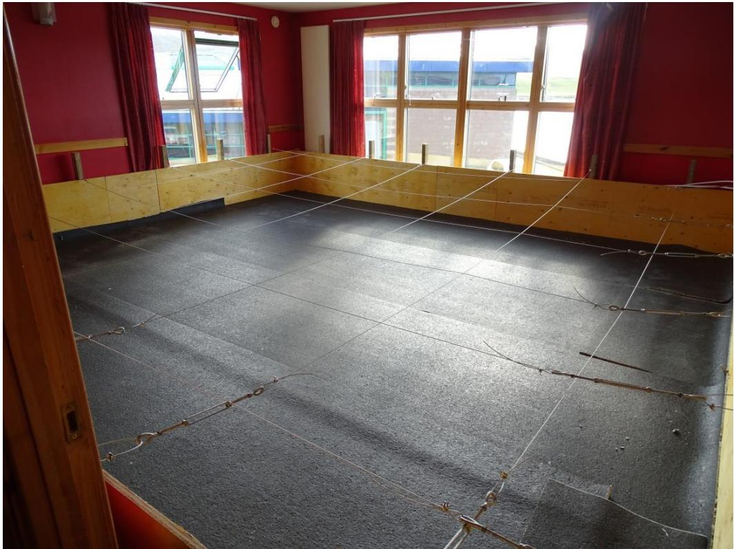
**Photograph 7** The tank under construction in the first floor lounge
