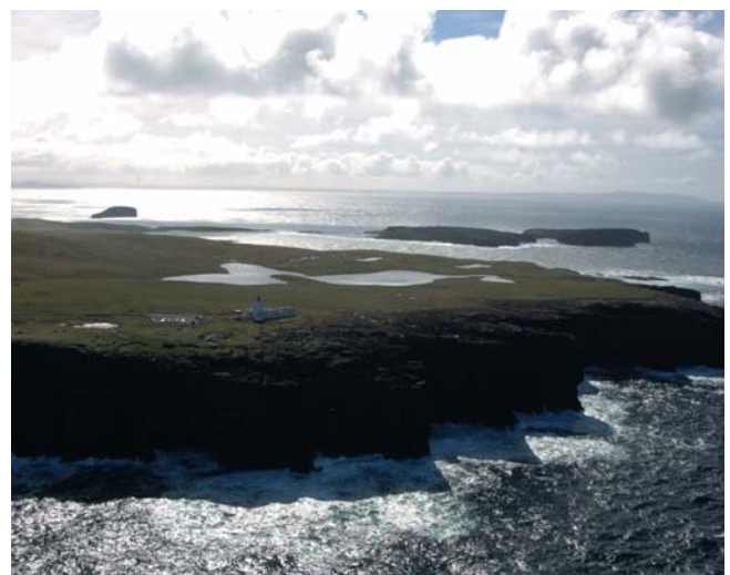
An aerial view of the lighthouse at Eshaness
