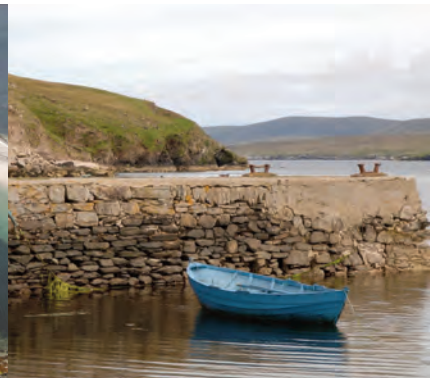
Pier at Yell Image courtesy of Promote Shetland
