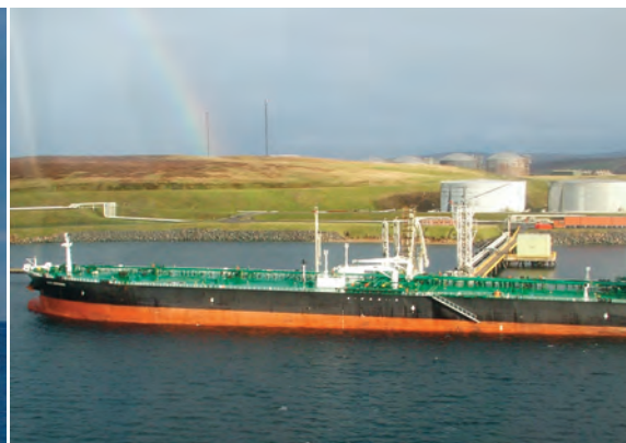
Sullom Voe Terminal Image courtesy of Stephan Hennig
