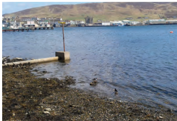
Waste pipe, Scalloway Image courtesy of Christina Kelly
