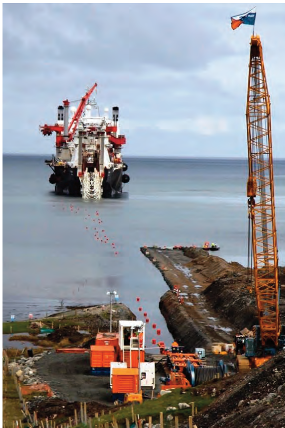
Solitaire, pipe laying vessel Image courtesy of Sheila Keith
